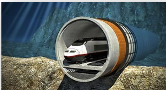
Tunnel immergé © Les Echos.fr
